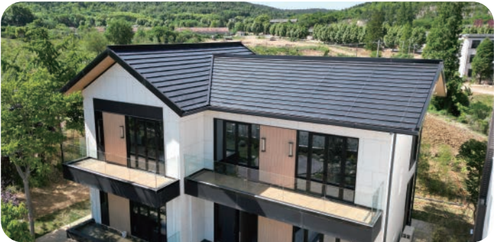
10.7KW Location: Anhui, China Date of installation: 2024 Project type: Residential - BIPV
