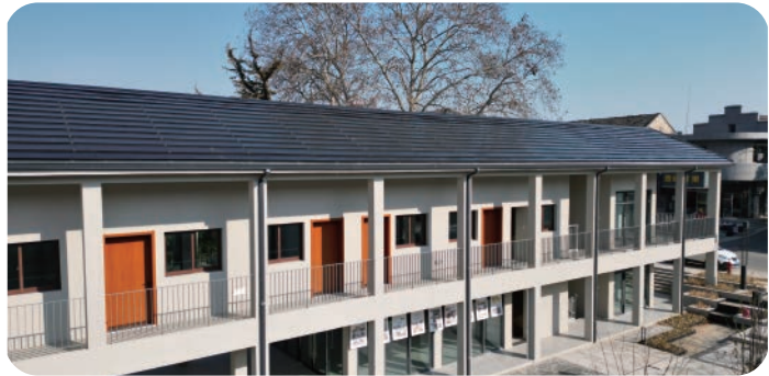
31KW Location: Nanjin, China Date of installation: 2023 Project type: Residential - BIPV
