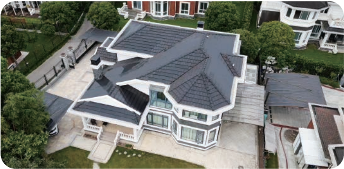
21KW Location: Shanghai, China Date of installation: 2023 Project type: Residential - BIPV
